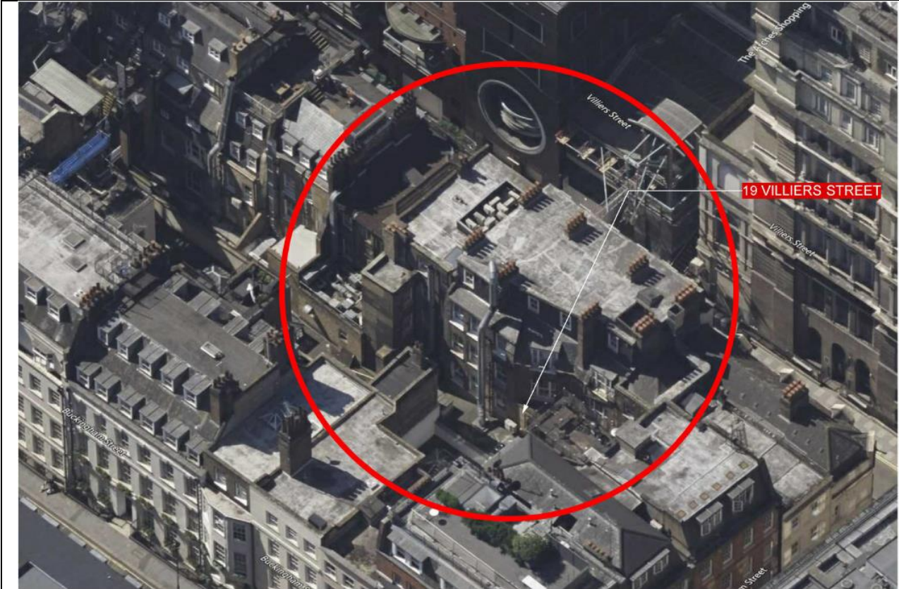
Rear of 19 Villiers Street (Aerial view)
