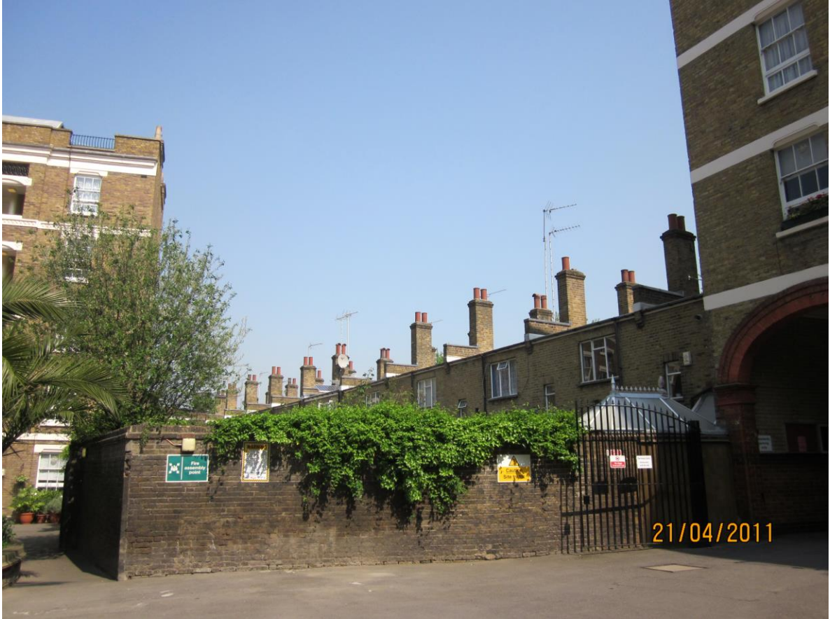
Rear elevation viewed from Lumley flats forecourt
